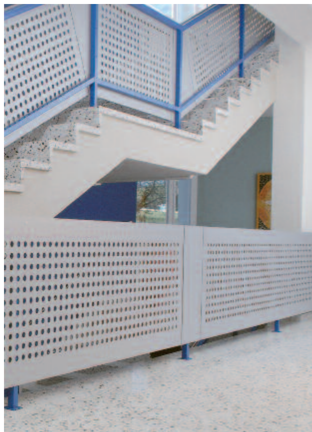
Staircase railing-enlarged holes in Max Alucompact42
